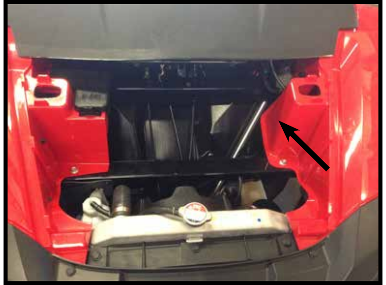
“Figure 7” Contactor Location
