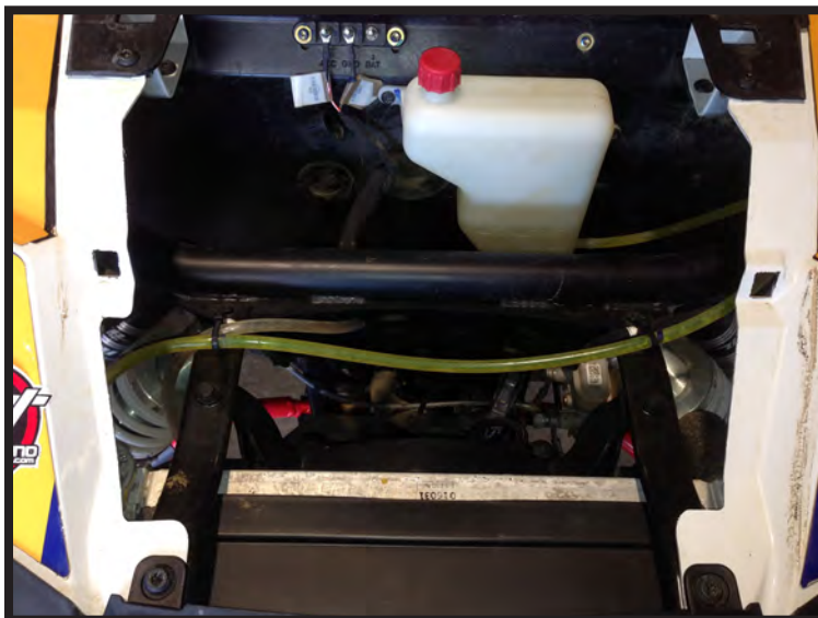
“Figure 12” Contactor Location (Located under the hood.)
