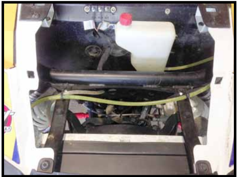
“Figure 11” Contactor Location (located under the hood)
